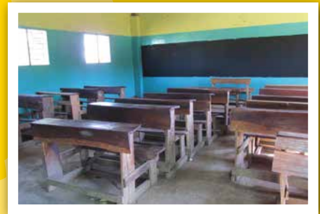
The classrooms start to take shape.
