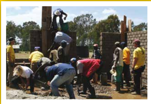
Mixing cement, back-breaking work in the heat.
